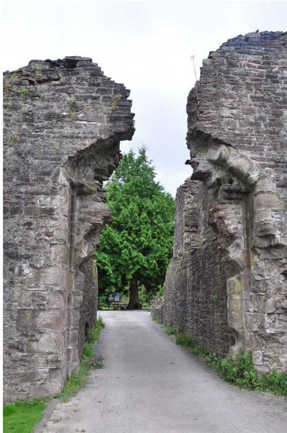
Original castle entrance Gatehouse
